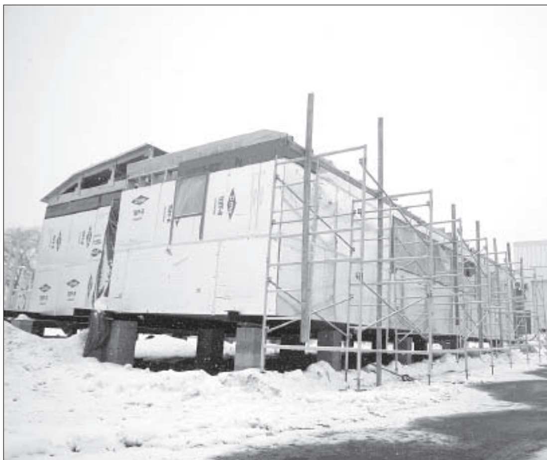
Joe McIntyre/staff photographer
